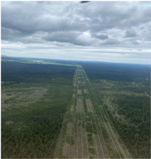
Figure 5. Fuel break linked to transmission line right-of-way
